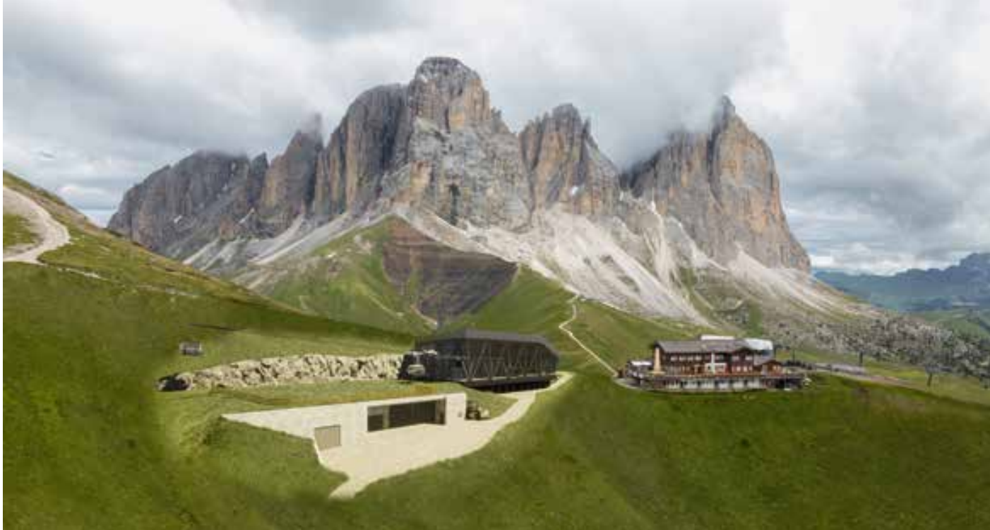
The top station is a glass structure on the side facing Canazei, while the rest of the station, as well as the cabin parking area, are underground to minimise environmental impact. © DOPPELMAYR
