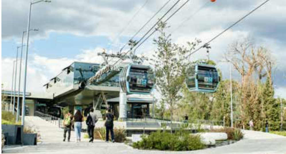
DOPPELMAYR has implemented Cablebús Lines 1 and 3 (pictured) in Mexico City, and another cable car is currently under construction in Uruapan. This is creating the most extensive urban cable car infrastructure in Mexico City – with a future total length of more than 50 kilometers, providing improved mobility for over 350,000 passengers daily. © DOPPELMAYR
