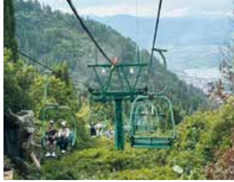
Xishan Scenic Area chairlift, before renovation. © BARTHOLET
