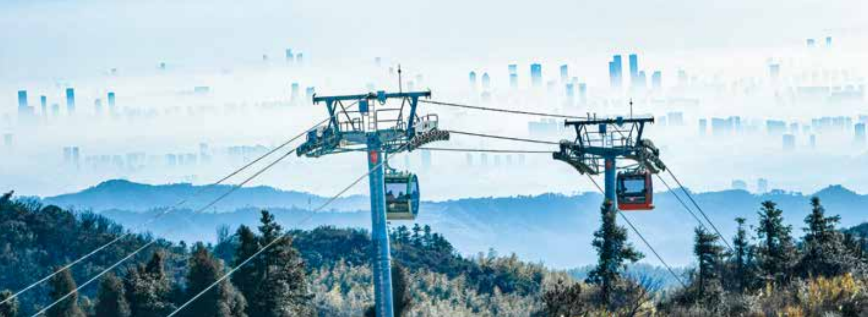
BARTHOLET's 8-person gondola in Meiling, Jiangxi, China, began operations at the end of 2025. © BARTHOLET
