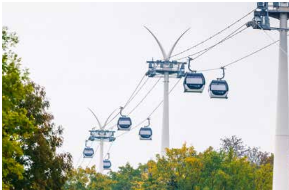
Câble C1 is a milestone in the field of urban cable cars. © Laurent GRANDGUILLOT / IDFM
