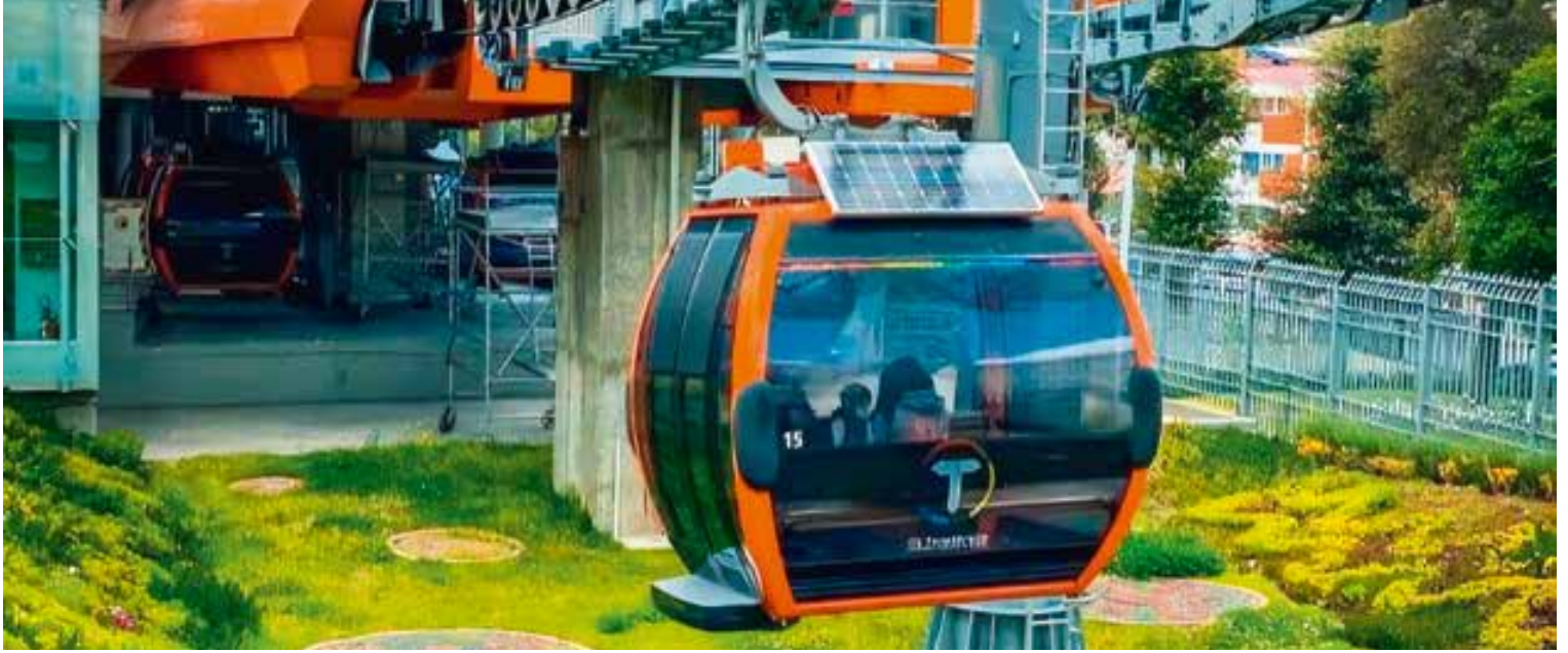
The management of “Mi Teleférico” in Bolivia is working together with international partners on a model for self-generation of renewable energy. © Mi Teleférico
