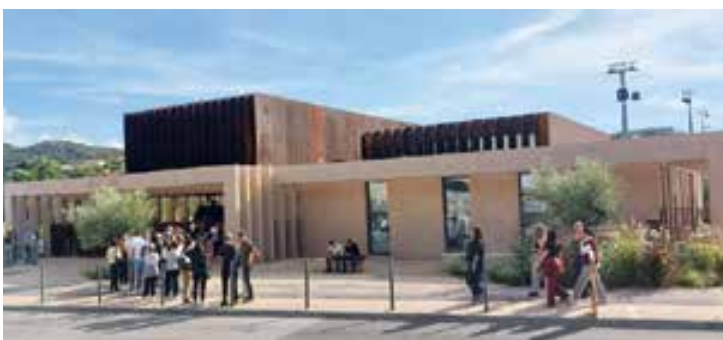
The stations are designed as multimodal hubs that interconnect various modes of transport.
