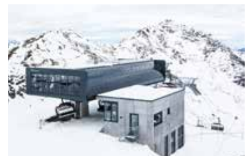
At the Waidoffen chairlift in Tirol, Austria, solar panels are directly integrated into the station buildings – a solution that is both aesthetically pleasing and functional.
