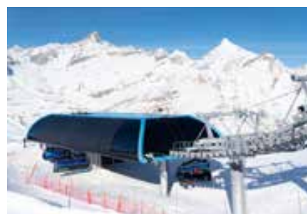
Solar modules are used on the Gifhittli chairlift in Zermatt, Switzerland. © Leitner
