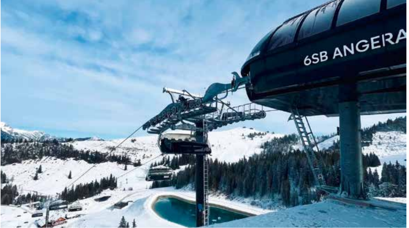
Sustainable use of materials is a key trend in the cable car industry. Shown here: the 6-person Jennerwiesen chairlift, relocated from Berchtesgaden to the Riedlkaralm at Dachstein West, now operating as the Angeralmbahn. © BBDS
