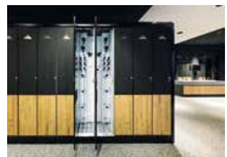
Fisser cable car valley station: heated lockers with drying systems in the ski depot.
