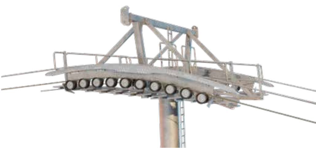
The optimised tower saddles reduce both the tower and foundation forces. Particular attention was paid to serviceability, such as roller removal without dismantling the bracket. © Barholet
