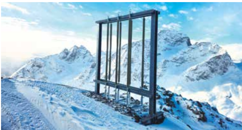
This is what a part of the thermosyphon looks like after installation.
