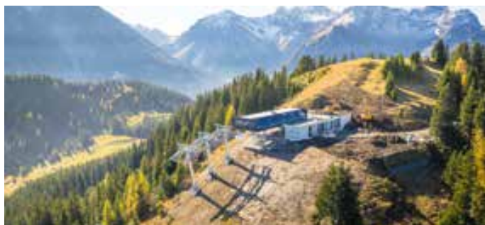
Operating in two sections, the 10-MGD Loischkopfbahn spans 1,829 meters, climbs 617 vertical meters in 7.9 minutes, and carries up to 2,500 passengers per hour with 60 cabins. © Roman Nöstler
