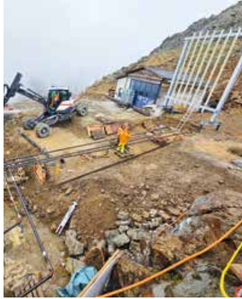
Permafrost-related ground ice and thermosyphon installation at Piz Nair, Engadin St. Moritz, Switzerland. © Engadin St. Moritz Mountains AG
