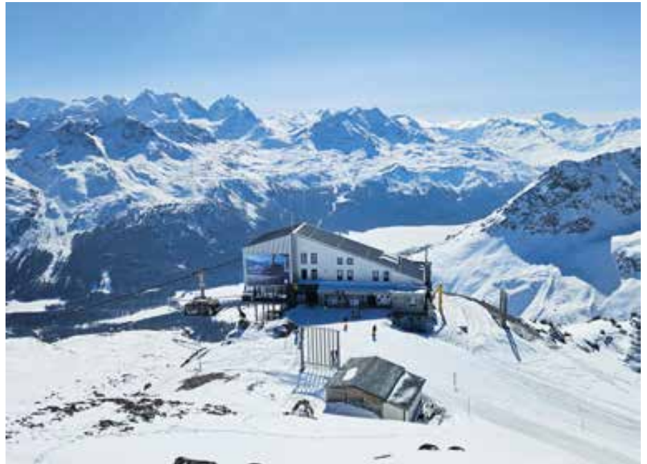
Thawing permafrost poses a serious threat to ski resorts: what often starts harmlessly with cracks in concrete or jamming doors and windows can later lead to the severe consequences. The Piz Nair mountain station in the Swiss Engadin was confronted with exactly this problem.
