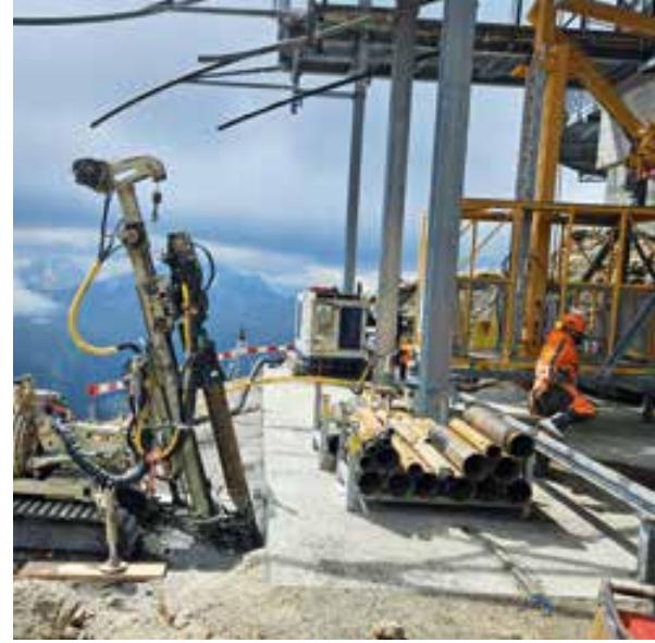
Permafrost-related ground ice and thermosyphon installation at Piz Nair, Engadin St. Moritz, Switzerland. © Engadin St. Moritz Mountains AG
