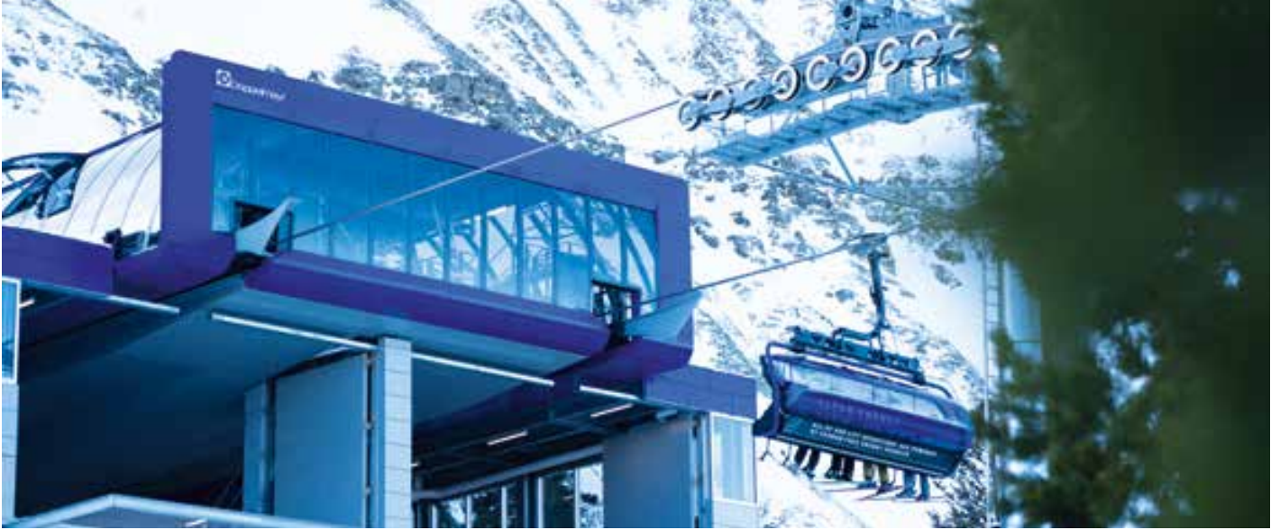
At an inclined length of 8,631 feet, Madison 8 now holds a record as the world's longest eight-place chairlift installation. © DOPPELMAYR
