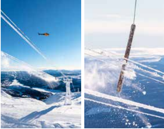
De-icing in Åre with the help of tree trunks and helicopters. © FB-Screenshot/Åre
