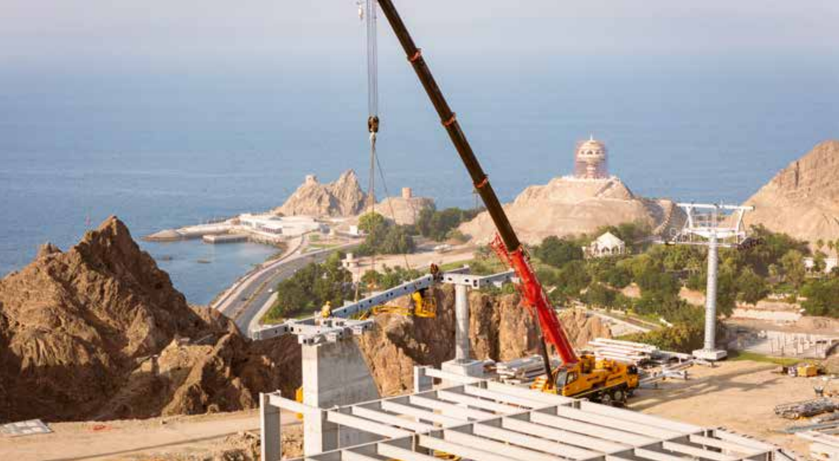
In Muttrah, the historic port city near the capital Muscat, construction of the new BARTHOLET cable car is progressing rapidly. It is set to boost tourism in the region while offering spectacular views. © BARTHOLET
