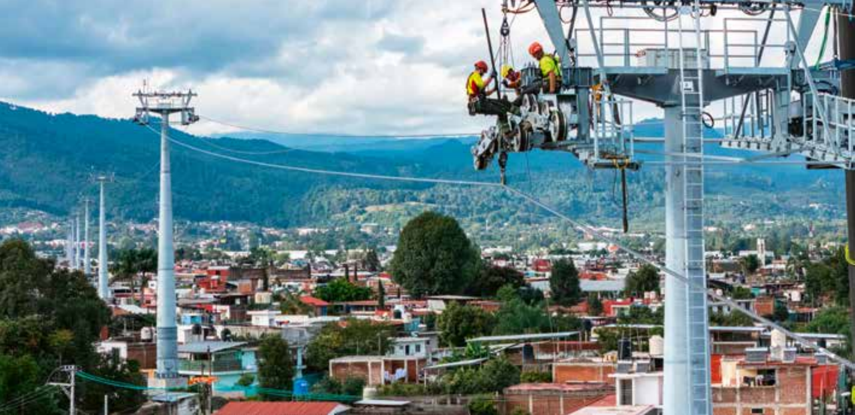
The 8.4-kilometer-long cable car in Uruapan will be the longest in Mexico upon completion. Two PERFORMA ropes with a diameter of 50 millimeters will allow the transport of 1,500 passengers per hour. © DOPPELMAYR MX
