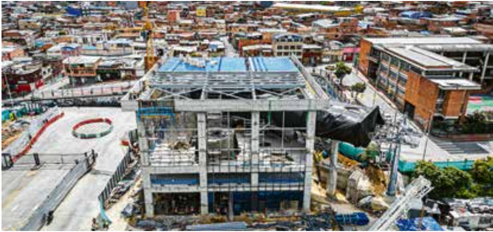
Construction work on the cable car in the San Cristóbal area. © Instituto de Desarrollo Urbano
