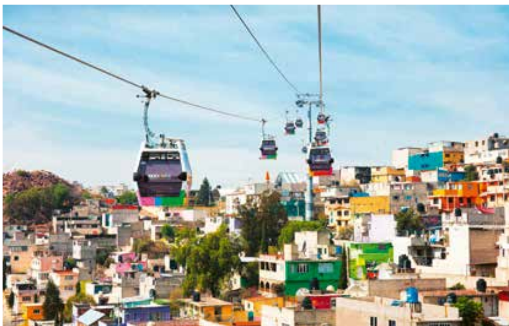
Linea Verde in Ecatepec (Mexico City) demonstrates what cable cars are capable of. © LEITNER
