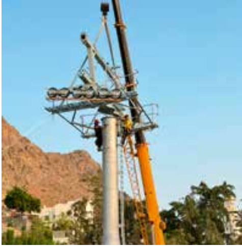
BARTHOLET's tallest towers, 71 and 87 meters high, are being built here.
