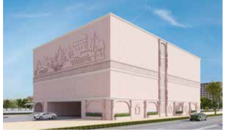
The cable car starts at the railway station of Ujjain. © NHLML
