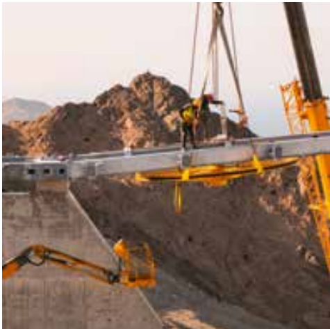
Work is now in full swing.
